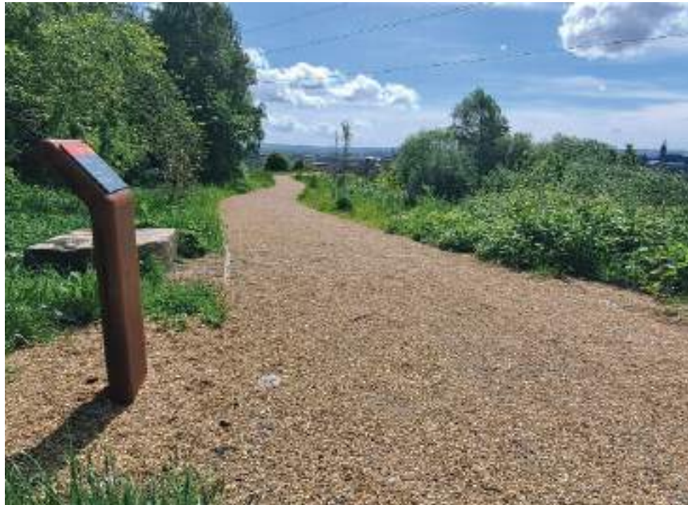
Self-binding gravel surfacing - Claypits - LUC Glasgow
