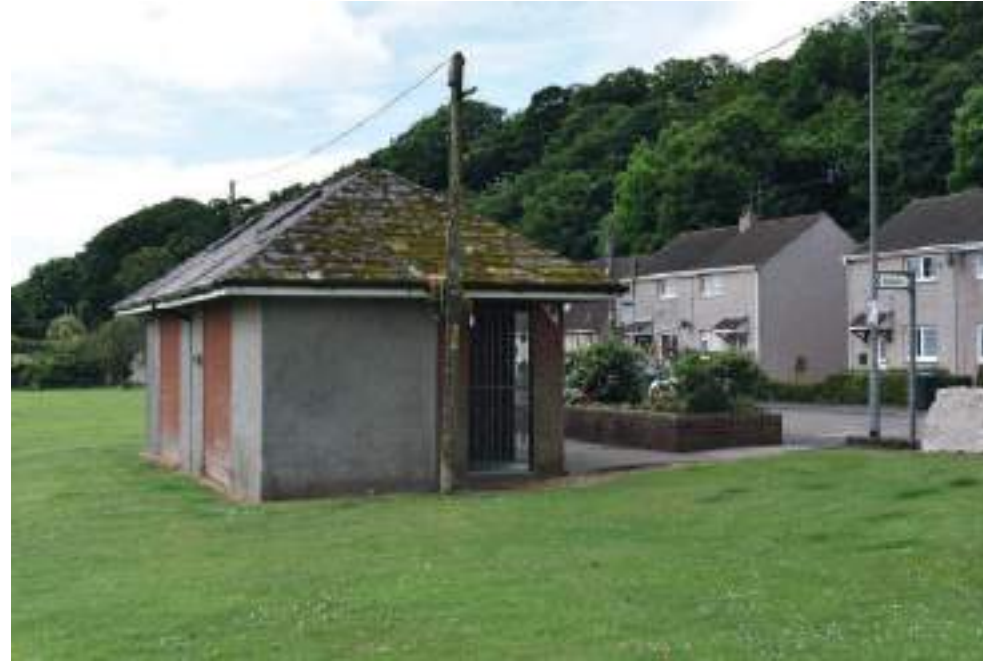
Image 02 - Public toilet near village main street
