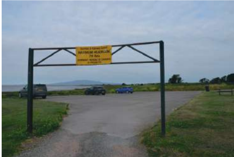
Image 01 - Car parking area and gate restriction
