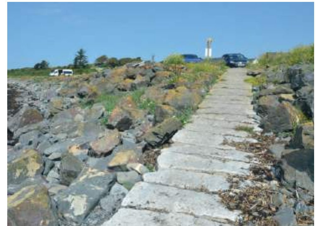
Natural stone ramped access
