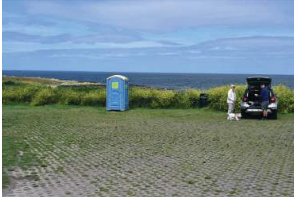
Image 01 - Matrix parking surface and toilet facilities
