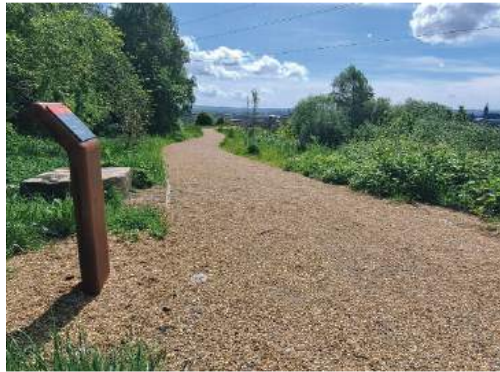
Self-binding gravel surfacing - Claypits - LUC Glasgow
