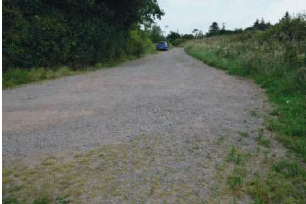
Image 01 - Car parking Area
