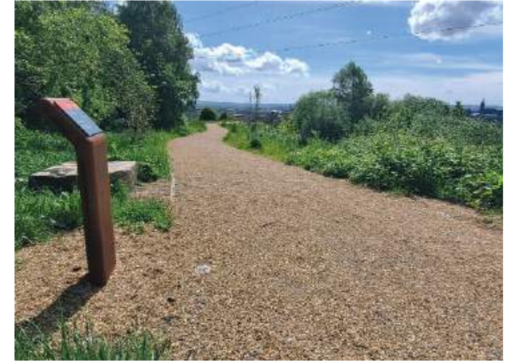
Self-binding gravel surfacing - Claypits - LUC Glasgow
