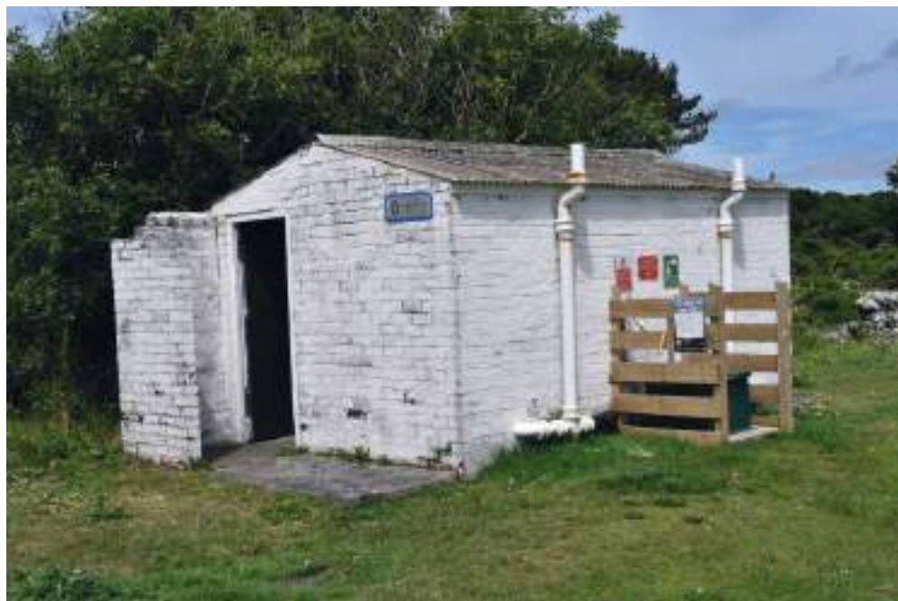
Image 04 - Public toilets with waste-water facilities for campervans
