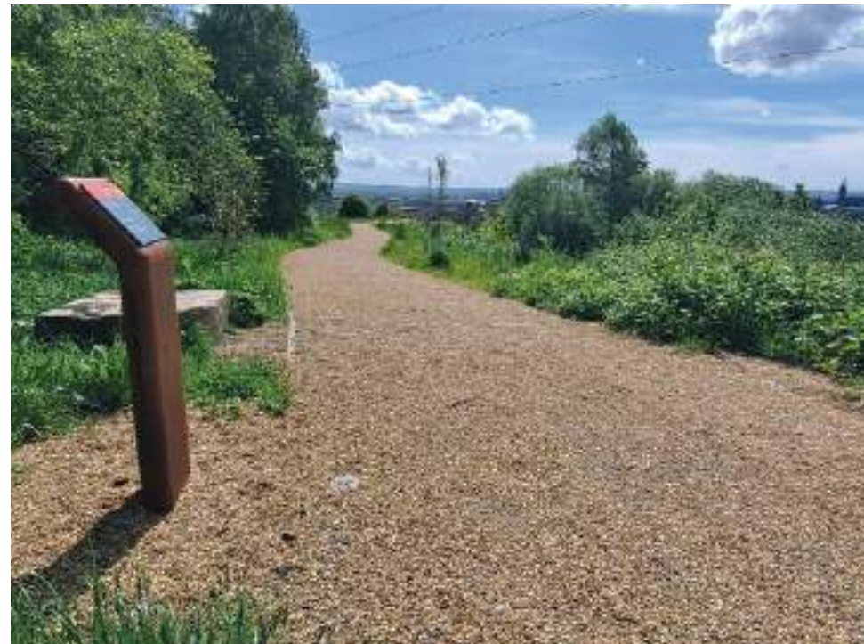
Self-binding gravel surfacing - Claypits - LUC Glasgow
