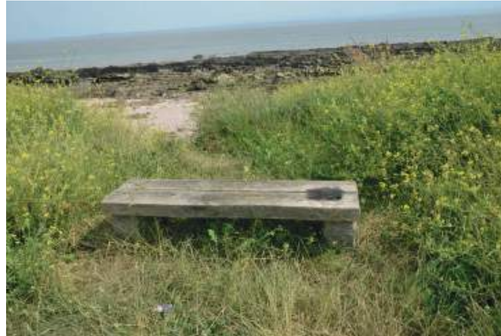
Image 02 - Seating area with damage
