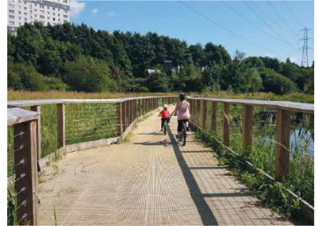
Boardwalk with tension wire balustrade - Claypits, LUC Glasgow
