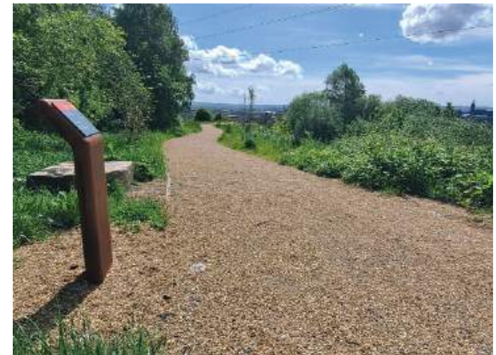
Self-binding gravel surfacing - Claypits - LUC Glasgow
