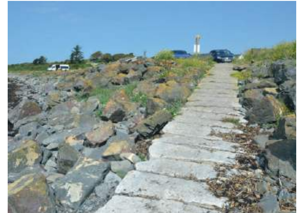
Natural stone ramped access
