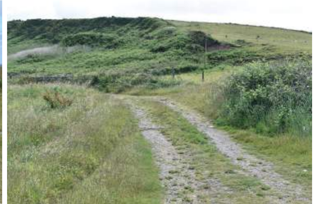
Image 03 - Site access track condition
