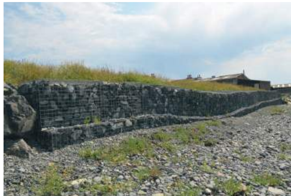
Image 05 - Gabion retaining wall
