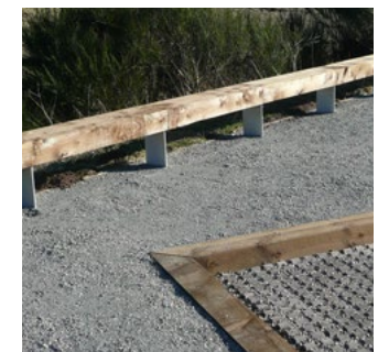
Galvanised Steel and Timber Knee Rail
