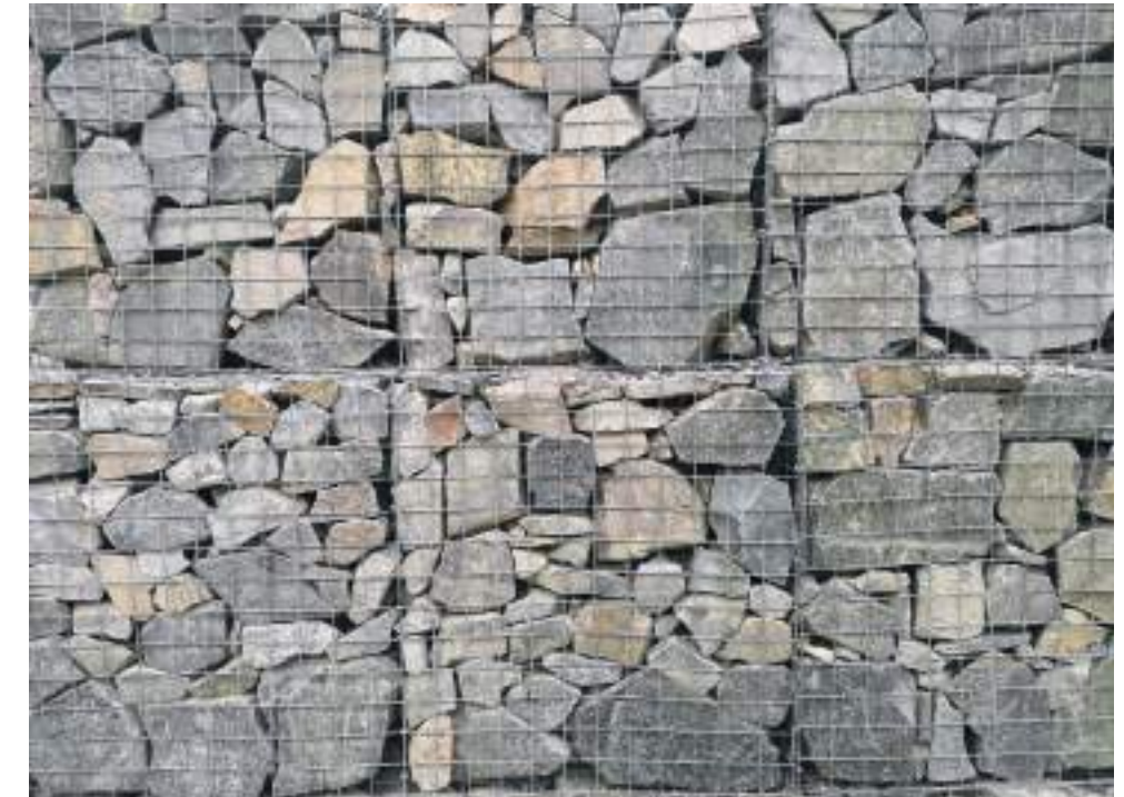
Hand faced welded mesh stone Gabion retaining wall
