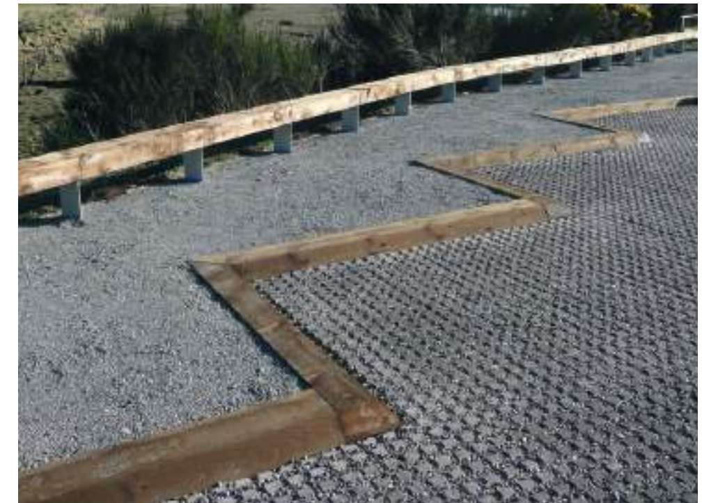
Timber knee rail and parking demarcation - Forvie Nature Reserve - LUC Glasgow
