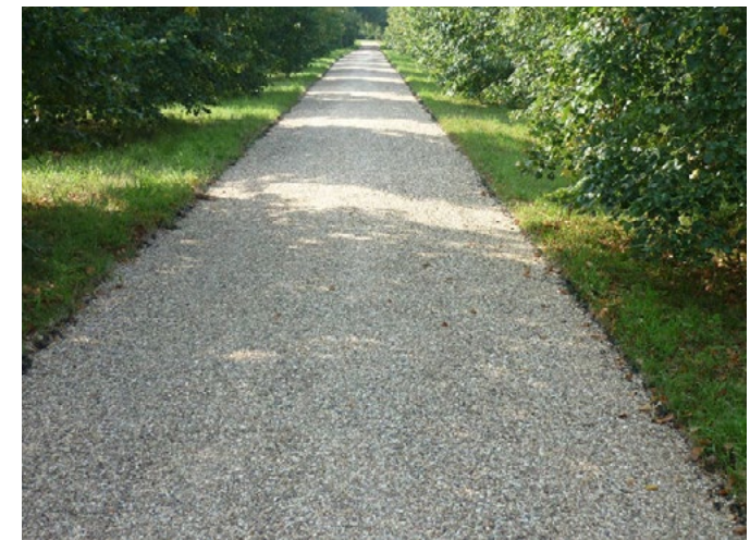
Bitumen Emulsion-Bonded Surfacing
