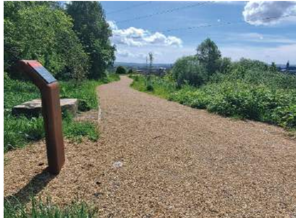
Self-binding gravel surfacing - Claypits - LUC Glasgow
