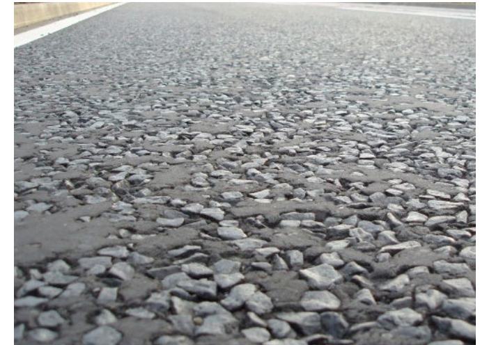
Hot Rolled Asphalt
