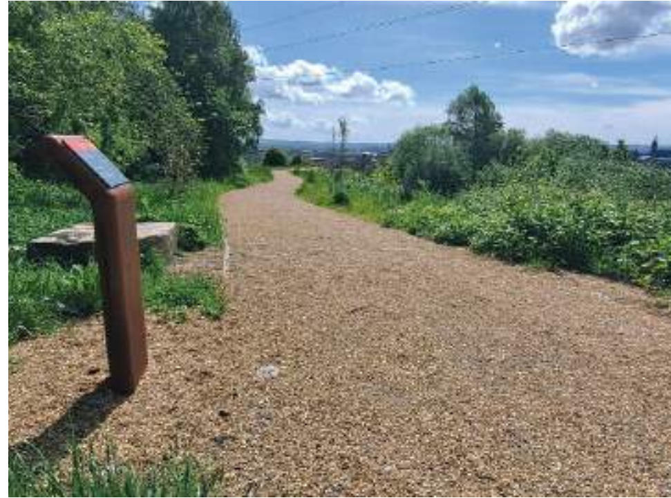
Self-binding gravel surfacing - Claypits - LUC Glasgow
