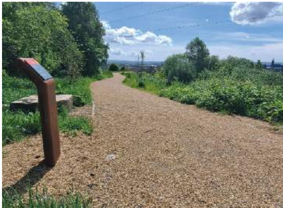
Self-binding gravel surfacing - Claypits - LUC Glasgow
