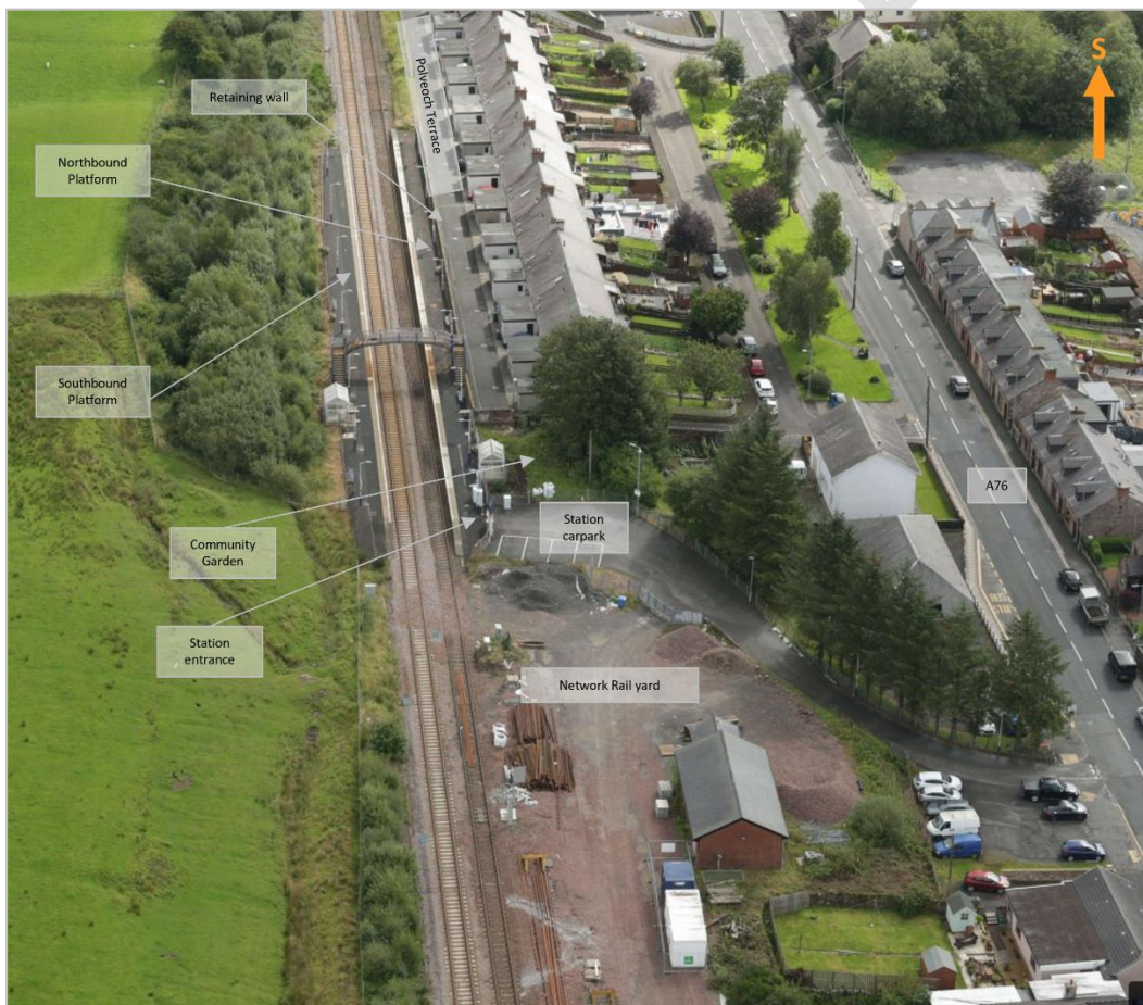
Figure 4.1: Kirkconnel Station - Ariel view (photo courtesy of Network Rail)
