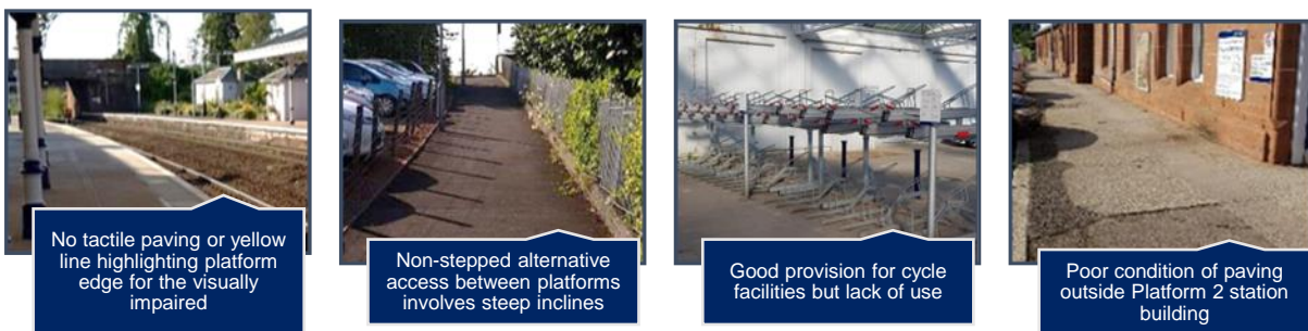
Figure 13: Audit Observations - Station Area
